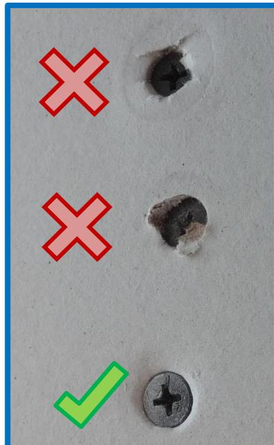
Screws which **break through the paper** must be **replaced**.
