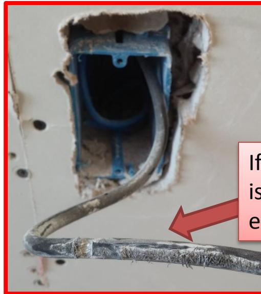
If *too much cutting surface* is exposed, bit will damage electrical boxes and wires.
