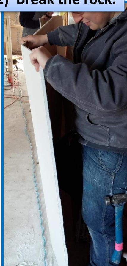
*With help,* pull the board away from the pile. **Push a knee into the back of the cut** to break the gypsum along the cut.
