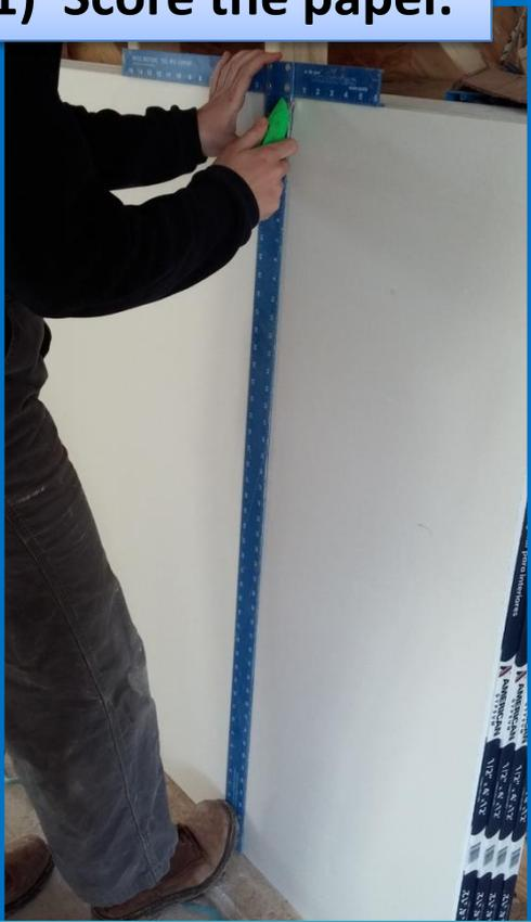
Hook the top lip of a **drywall square** over the top edge of piece. Use a foot to **push against the bottom** of the square so that it doesn't move as you cut along the edge. This ensures the cut is both **square and straight**.
