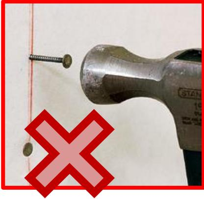
**Note:** Unless specifically called out *do not use nails to fasten drywall.*
